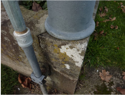
View of Typical Crack at Curb Corner
