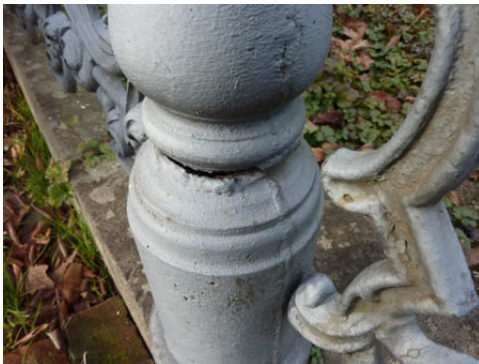
View of Crack at Gatepost 'G'
