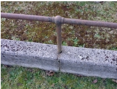
View of Rusted Out Pipe & Cracked Curb
