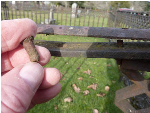
Countersunk Rail Fastener
