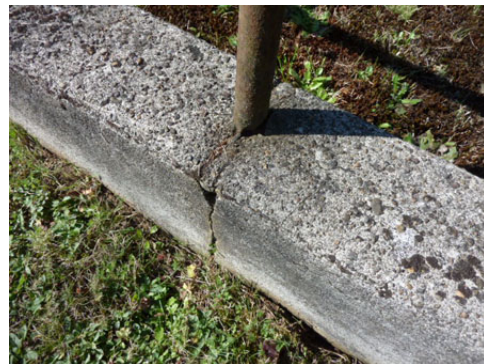
View of Typical Rust Damage at Posts
