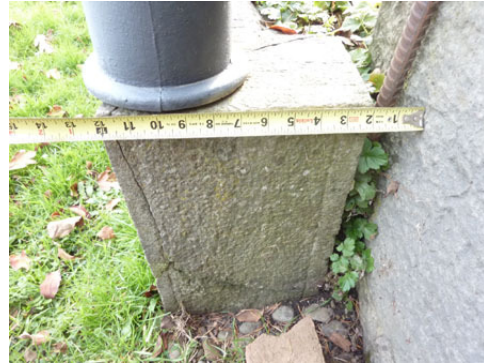
View of Misalignment at SE Corner of Vault
